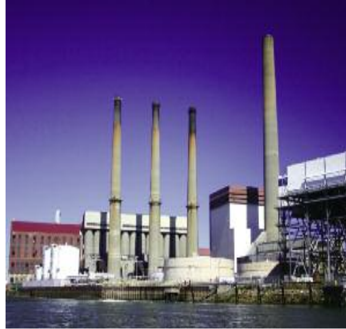
Siemens is uniquely equipped to handle all of the treatment solutions that power plants require.
